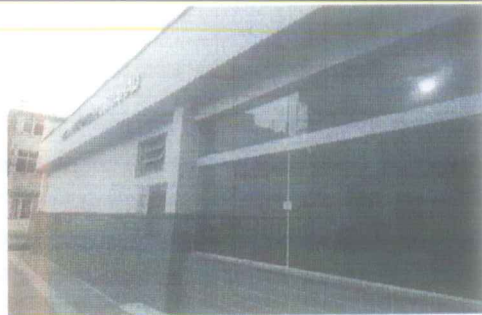
IMAGEM 4: E.M. JOSE MIGUEL MUAHAD LOCAL: FACHADA PRINCIPAL
